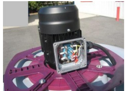
18. Wire the motor correctly according to your voltage.
