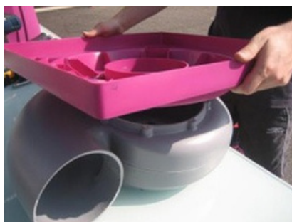
10. Place the roof curb base on the fan housing.
